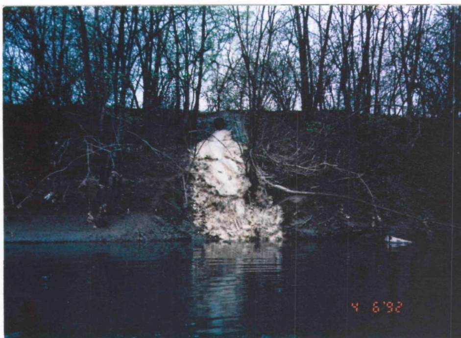
Plate 5. Discharges to Mill Creek from industrial activities. Top Photo: Silt laden discharge from Rack Sand and Gravel operation to Mill Creek in the concrete channel area. Bottom Photo: Cement discharge to Mill Creek from Plainville Concrete upstream from Clark Road. The concrete discharge had dried at the time of this photo.
