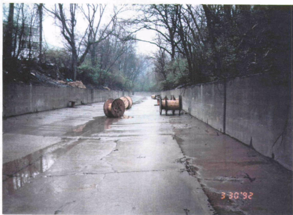
Plate 7. Large cable spools dumped into the channelized section of West Fork from a near by company.
