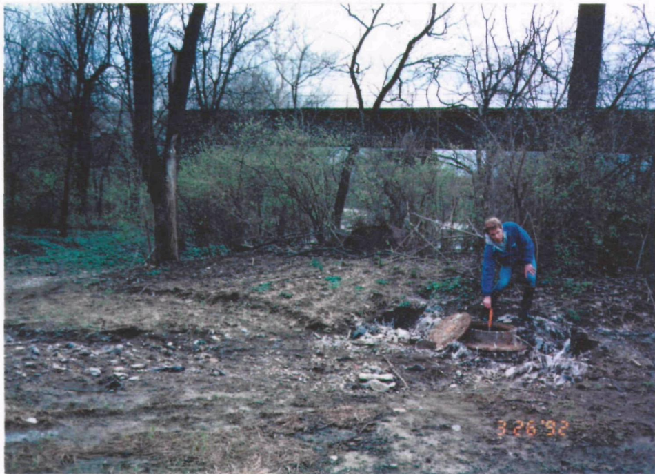
Plate 2. Sewer overflows in the Mill Creek basin. Top Photo: Raw sewage discharge to Mill Creek from broken sewer line cleanout at Windisch Road. Bottom Photo: Sewage solids trail leading to Mill Creek from an open manhole at the confluence of Mill Creek and Cooper Creek.
